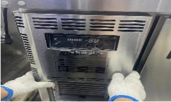
C. Remove the mech cover
