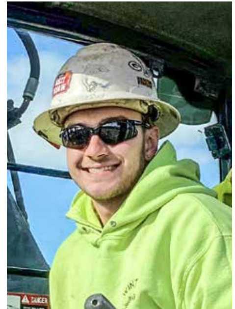
ON THE JOB for Winters Excavating in Brimfield at the Fire Station Project is Tyler Sharnsky.
