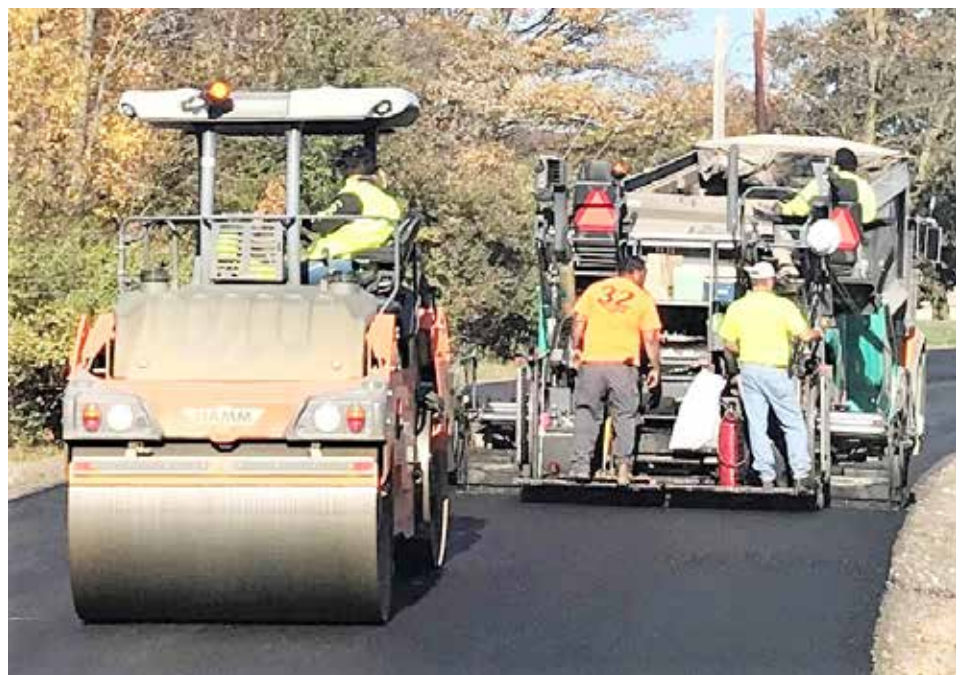
RESURFACING by Strawser Paving on Bixby Rd. in Groveport.
