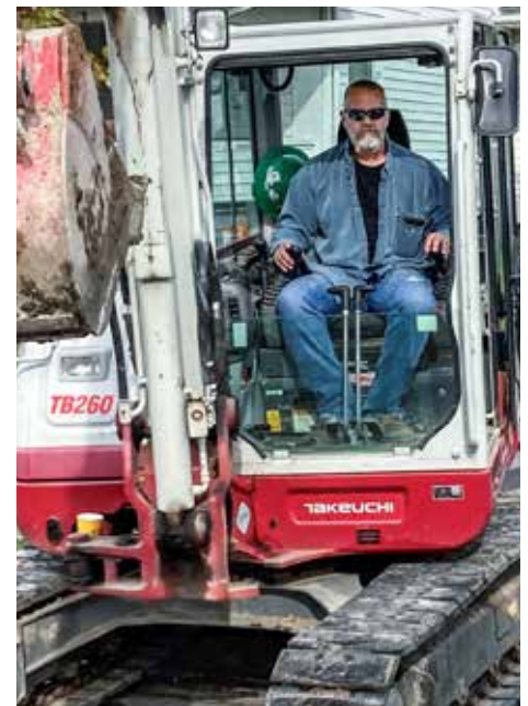
OPERATING an excavator in Springfield for Kinnison Excavating is Gary Burke.
