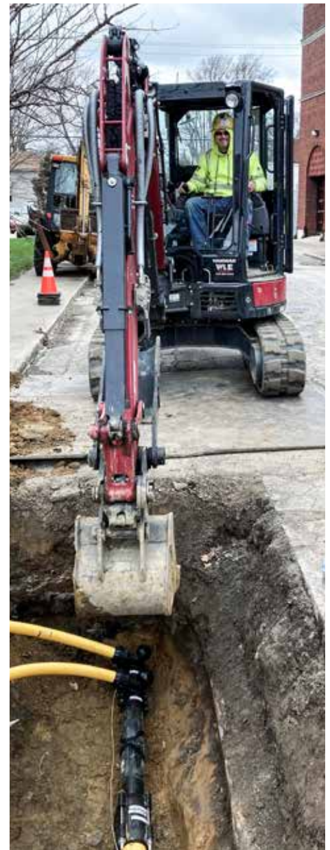
ON THE JOB for ASW Pipeline in Conneaut is Dave Lesperance.
