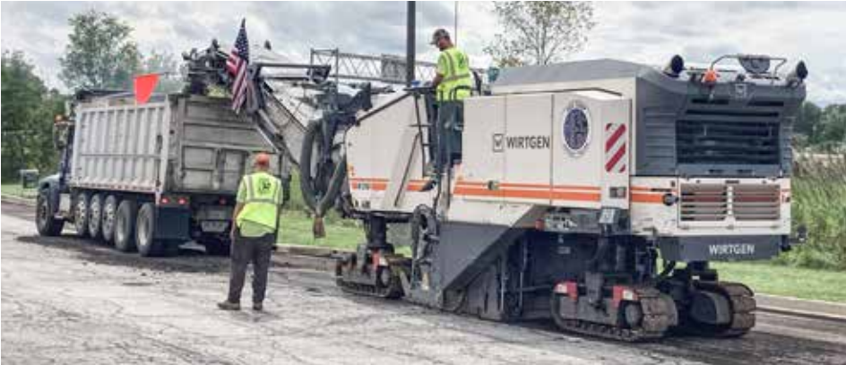
MILLING the Giant Eagle parking lot in Elyria for NES is Anthony Campbell.
