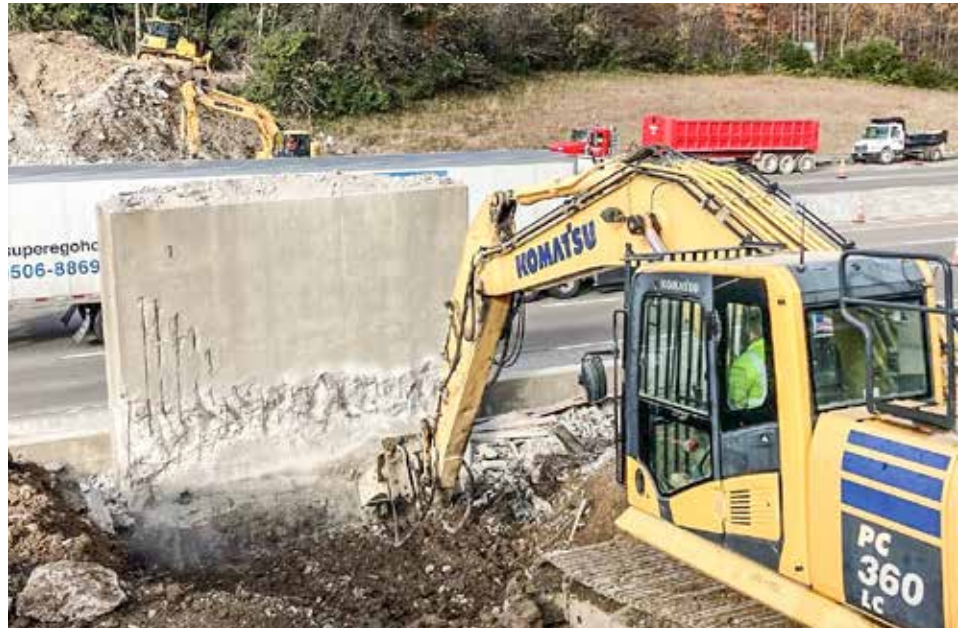
DEMOING a abandoned railroad bridge in Vandailia is Eagle Bridge.
