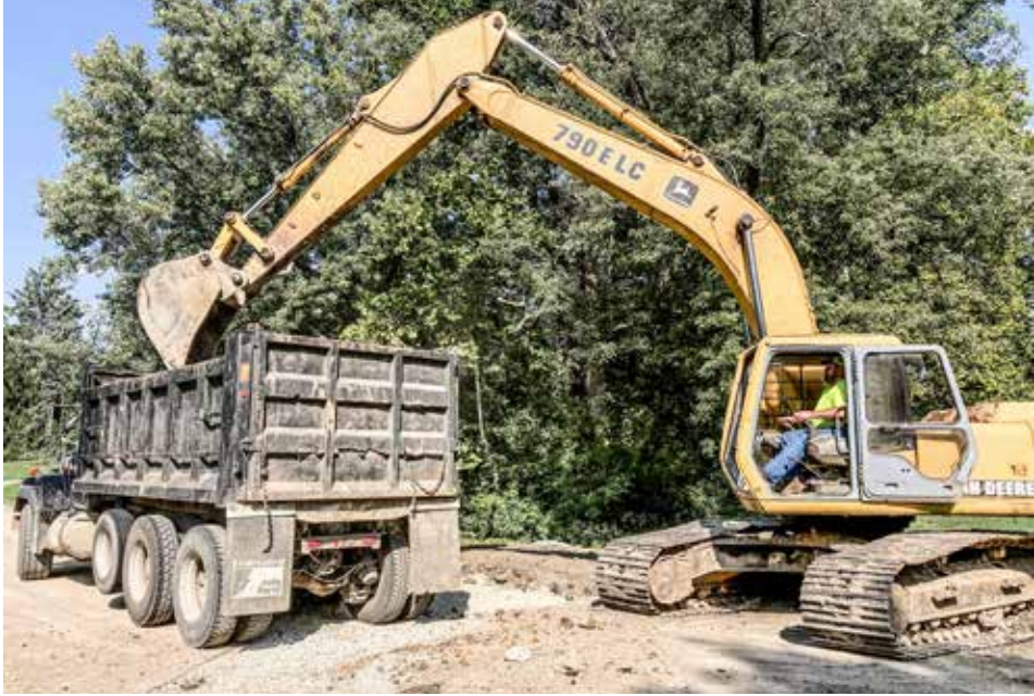
OPERATING an excavator for W.G. Stang in Vandailia is Richard Robinson.
